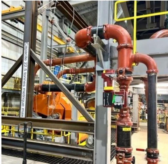
WHIMS rubber-lined piping (left); gate valves (right)
