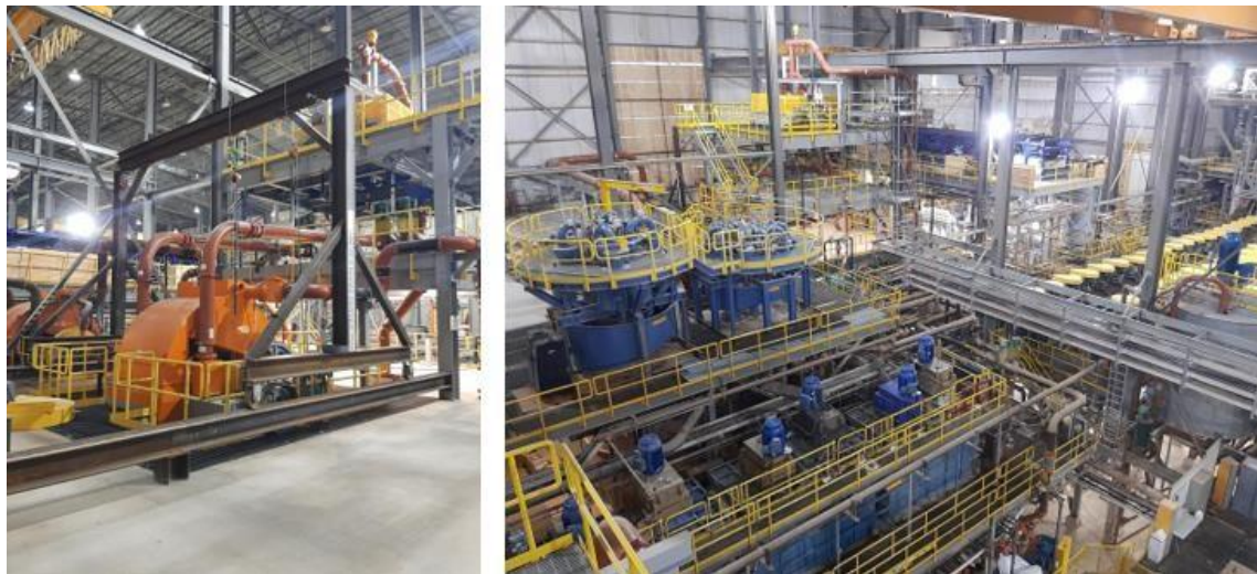
New WHIMS (left) and desliming area (right)
