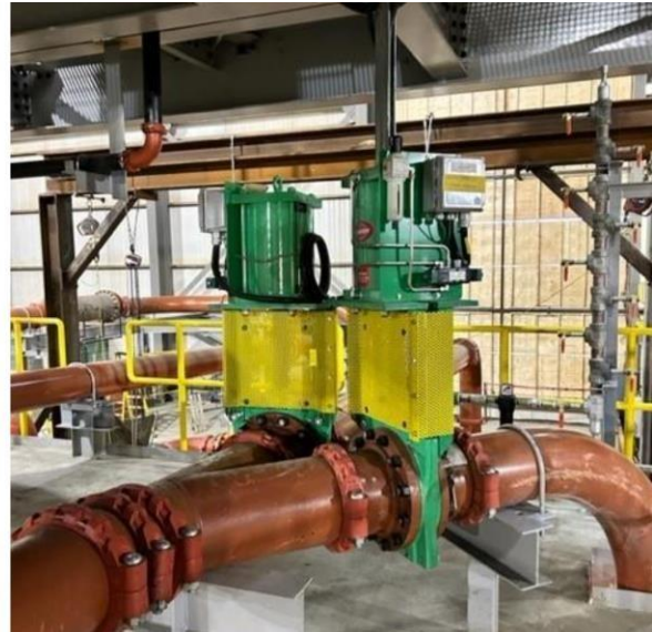
WHIMS rubber-lined piping (left); gate valves (right)
